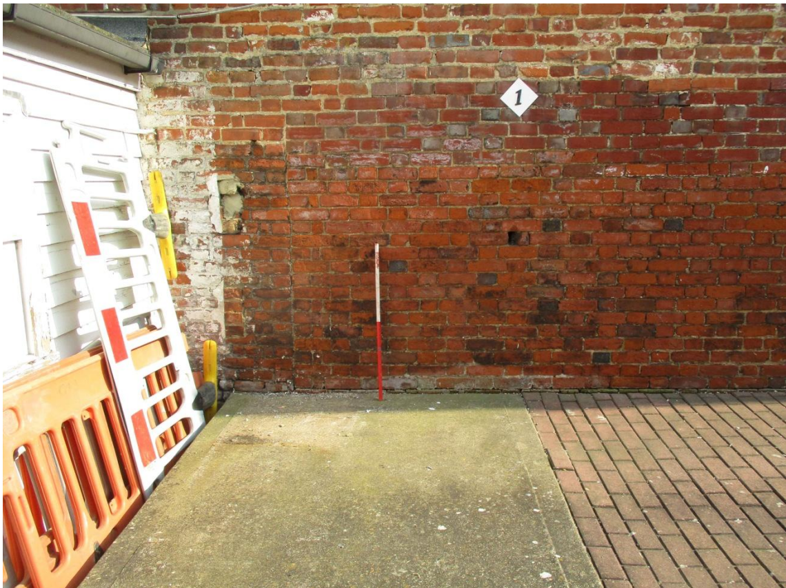
Plate 3: Looking north-east at Trench 2 prior excavation
